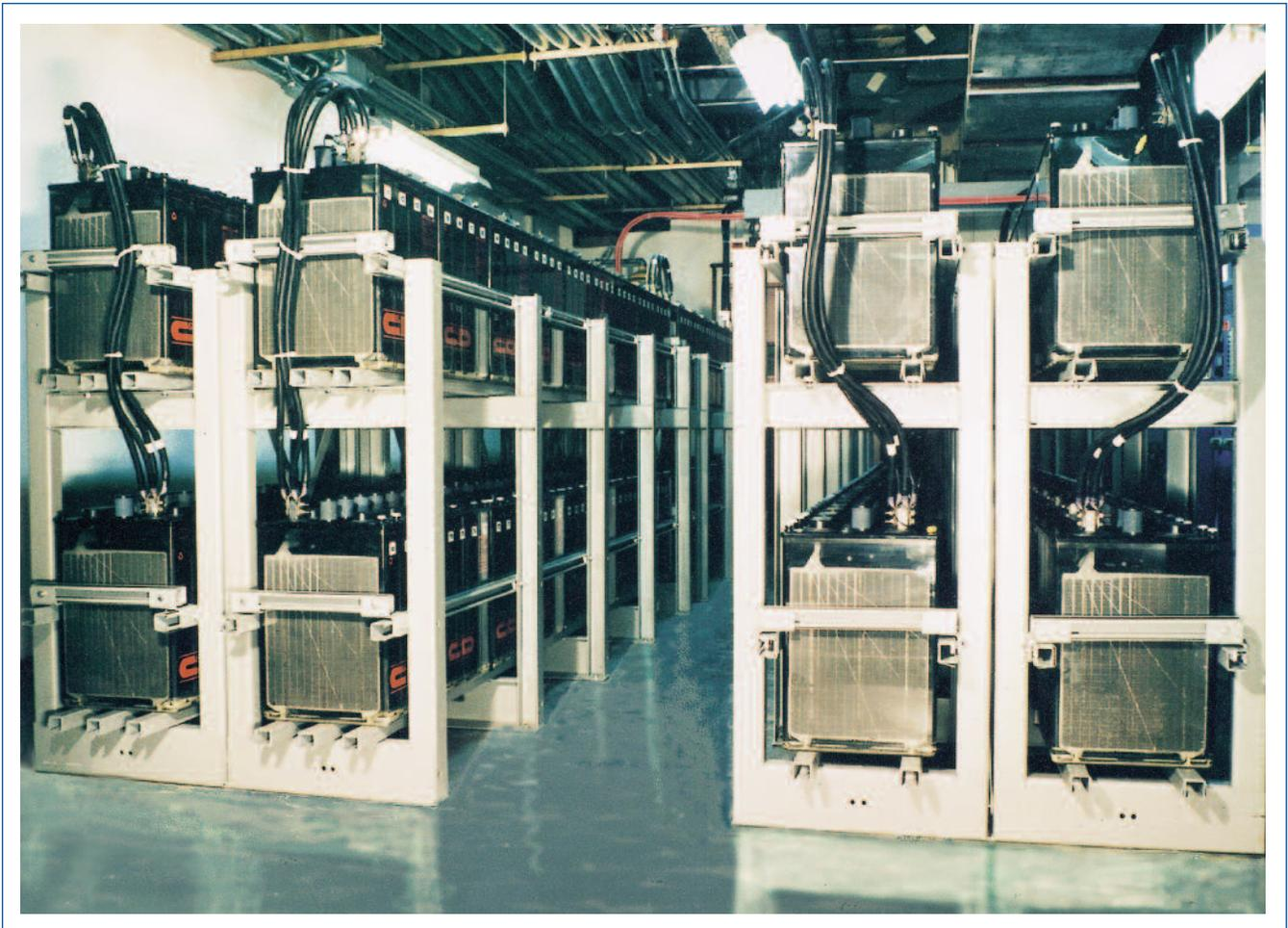
Shown: L-Series, 2-tier, EP, painted rail, back-to-back installation, with standard 2-rail and optional third (center) support rail.
